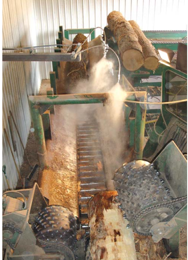
2-3 nozzles are mounted around the debarker to knock down the fine dust in the air. In addition, moisture on the logs will make it easier to turn the logs over.
